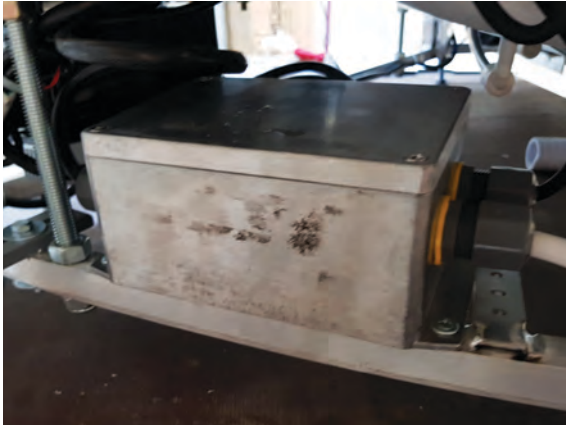
1. Electrical junction boxes
